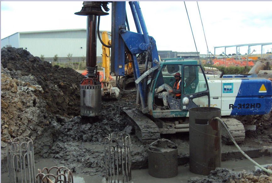
Drilling the 900dia piles under water pressure and polymer
