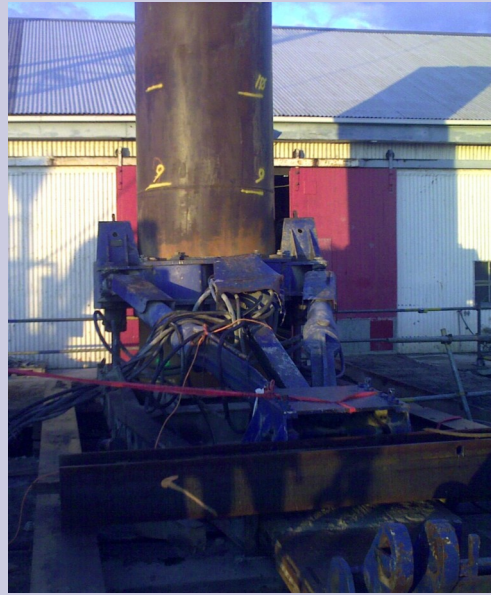
Oscillating 1500 dia Casing through the basalt
