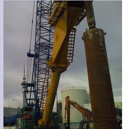
Screwing 900 dia casing with crane and drill table
